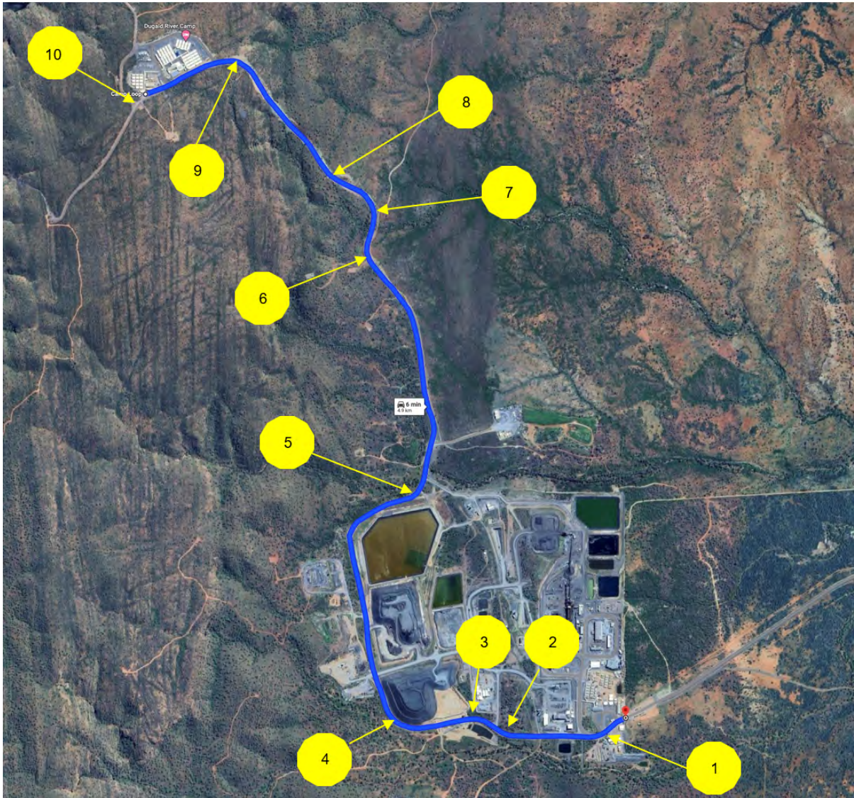
Figure 50 - Site Access Road
