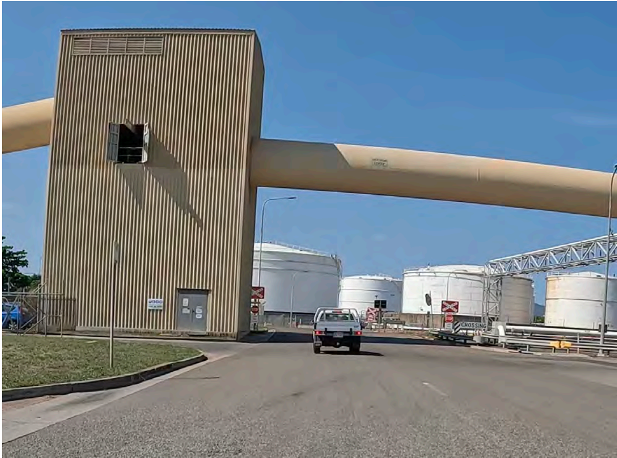
Figure 9 - Overhead conveyor on Centenary Drive
