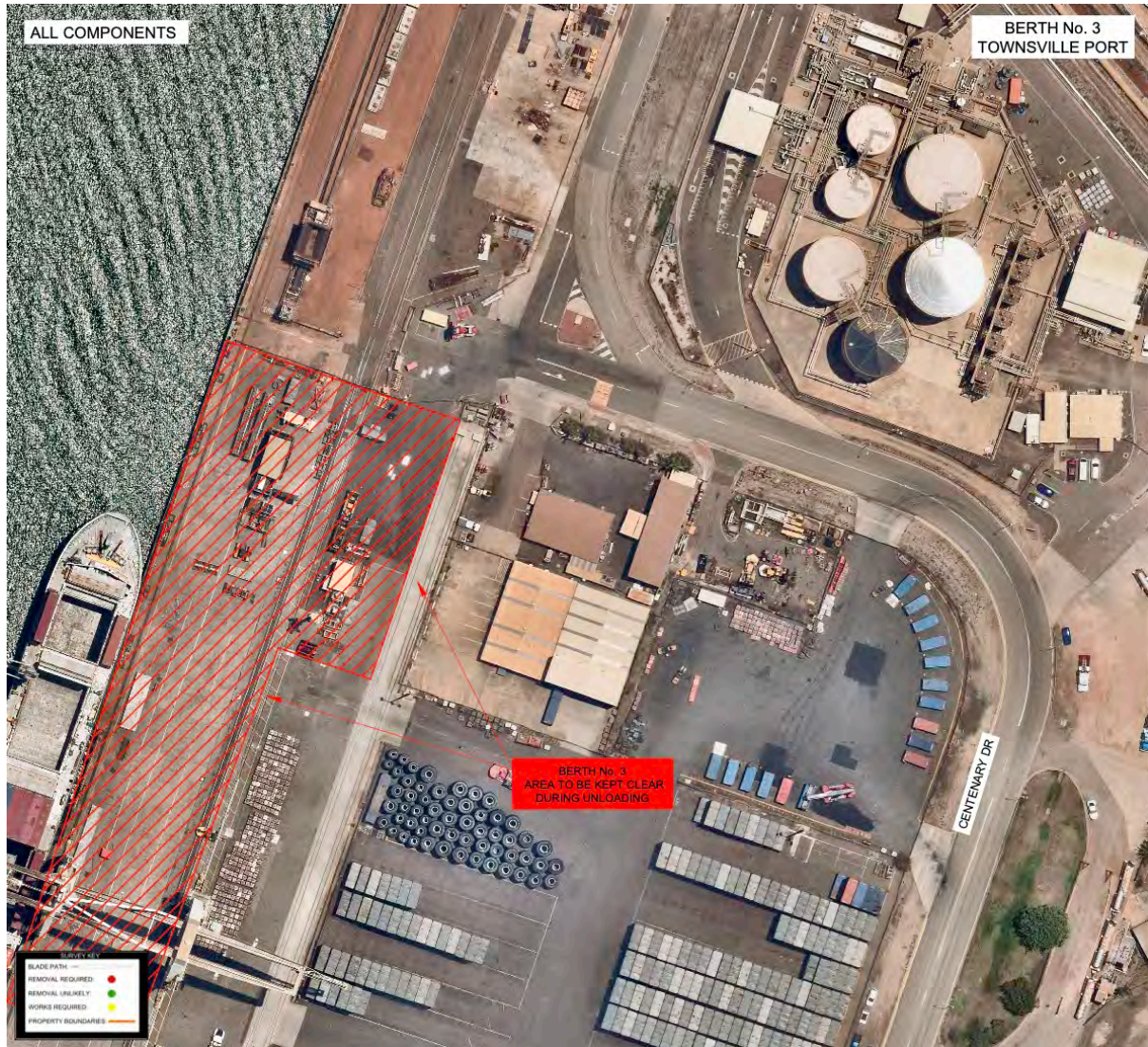
Figure 5 - Townsville Berth No. 3
