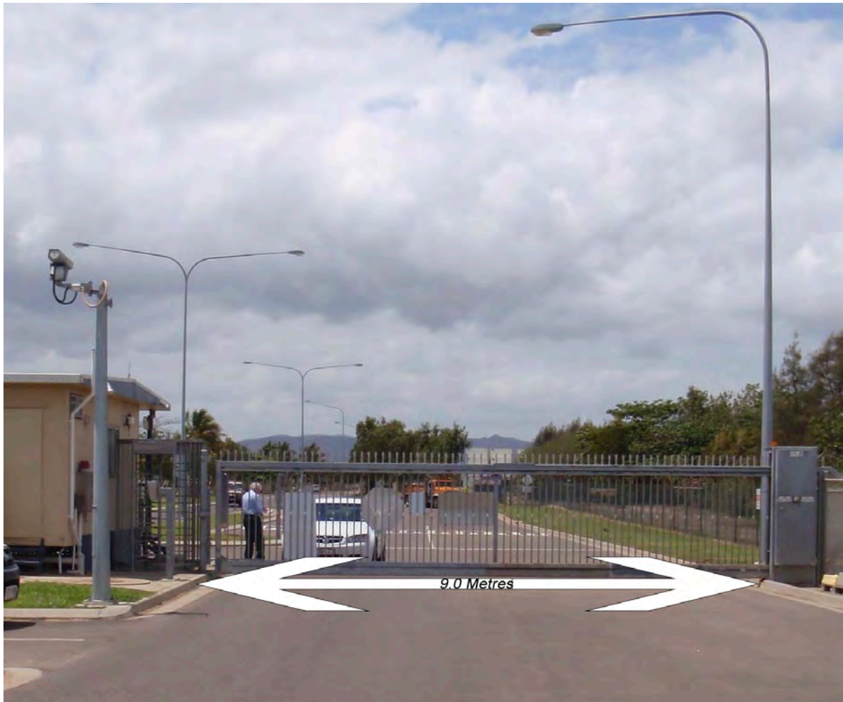
Figure 15 - Port access gates on Benwell Road
