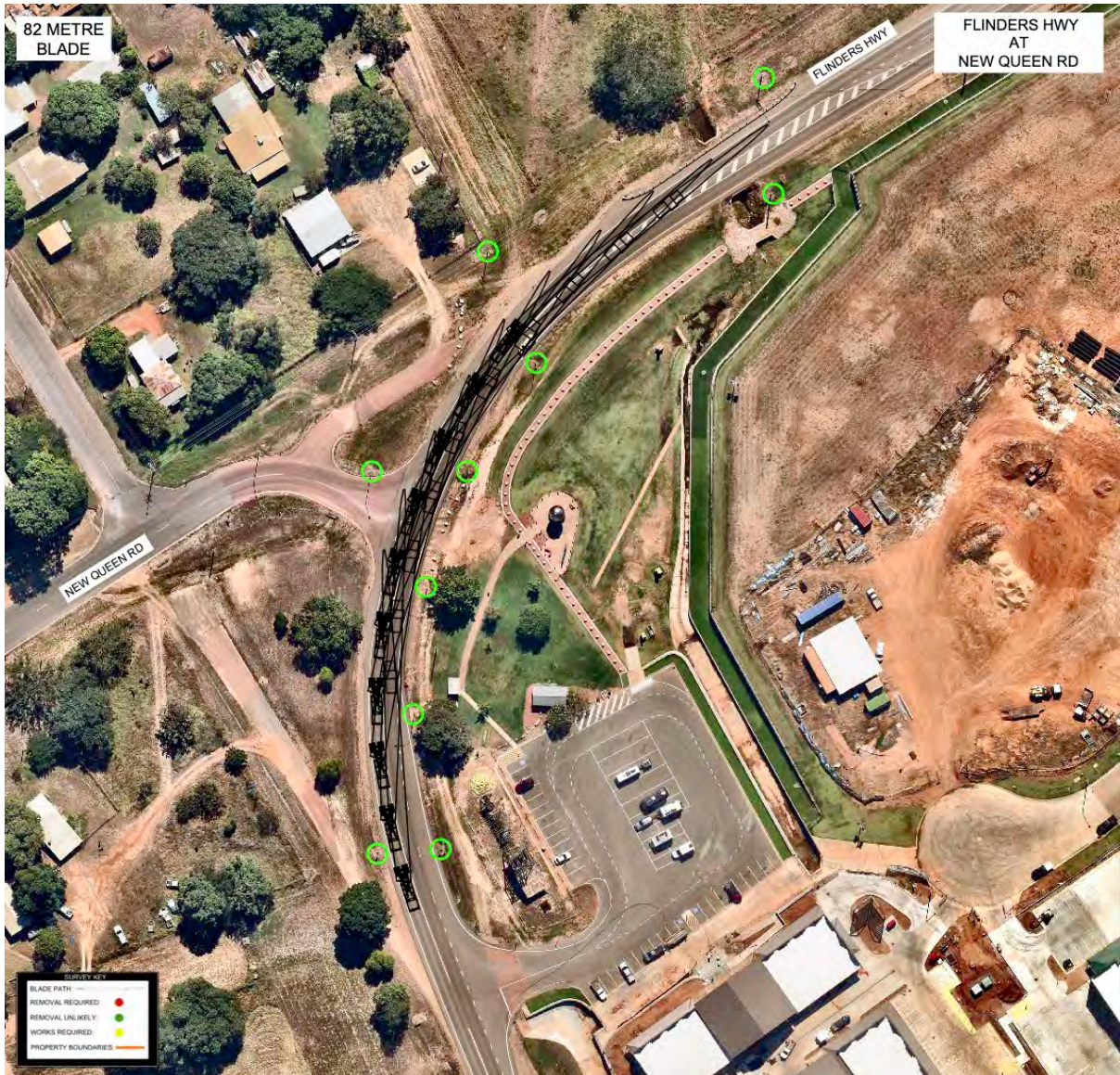
Figure 23 - LH bend on Flinders Highway at new Queen Rd
