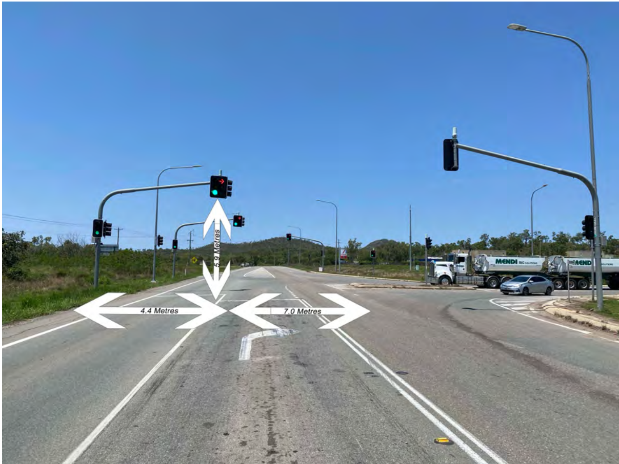
Figure 21 - Intersection of the Flinders Highway and Kiernan Drive
