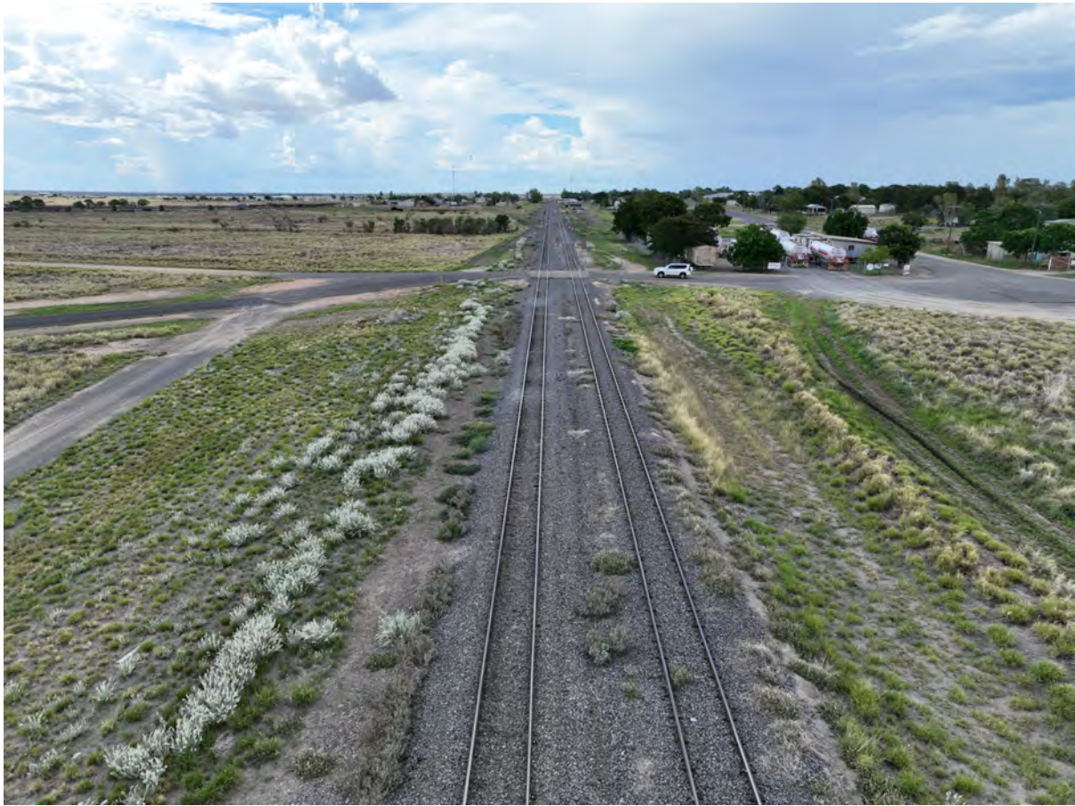
Figure 37 - Burke Street Over Rail Crossing
