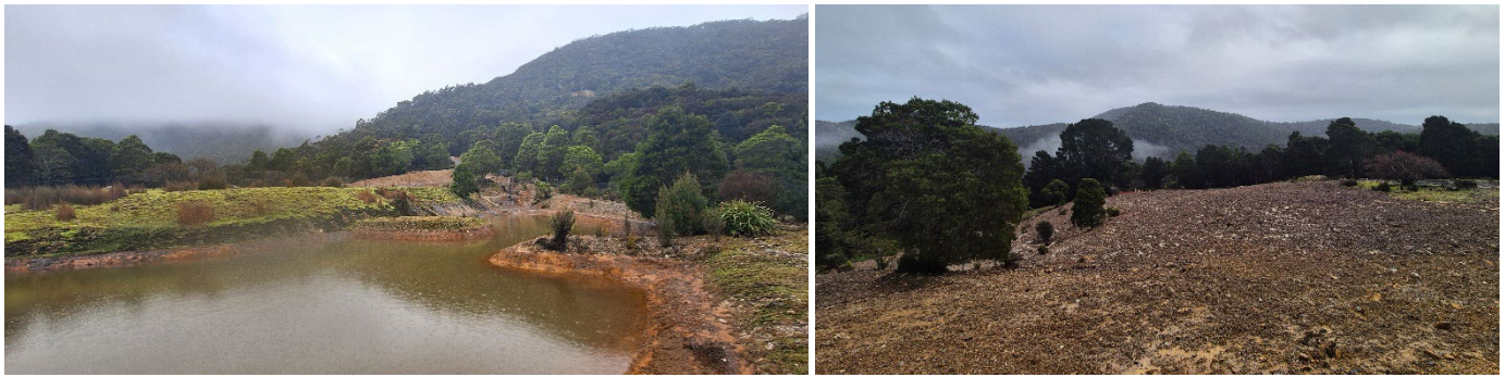
Figure 6. WSP before (left) and after (right) civil works have been completed in June 2026.
