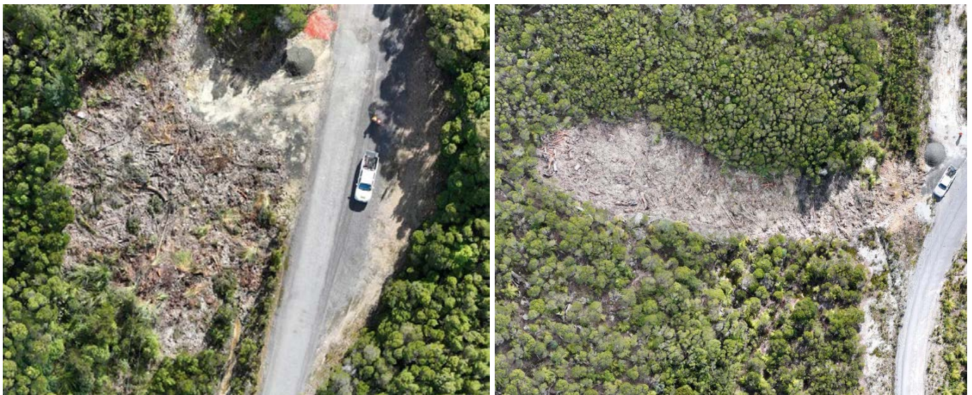
Figure 5. Two rehabilitated drill pads located along Mt Read Road as of September 2025.
