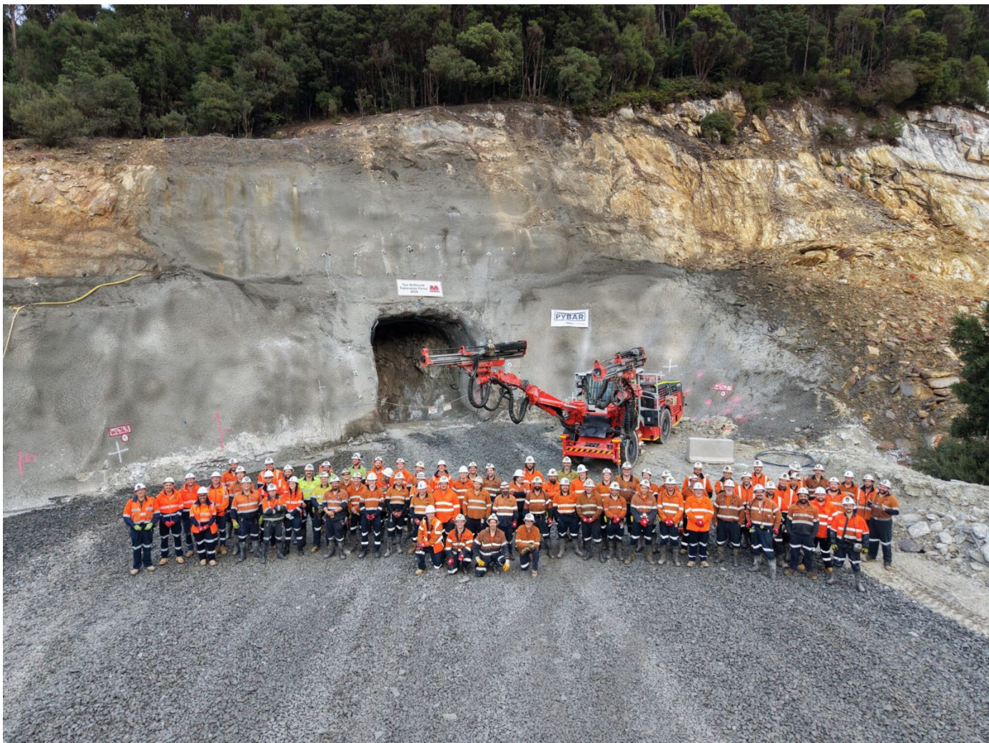
Figure 3. Cutting of the Tom McDonald Exploration Portal.
