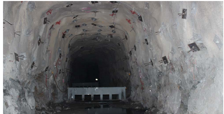
2014: Trial stoping program at Dugald River
