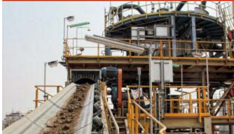
Process Plant, Kinsevere
