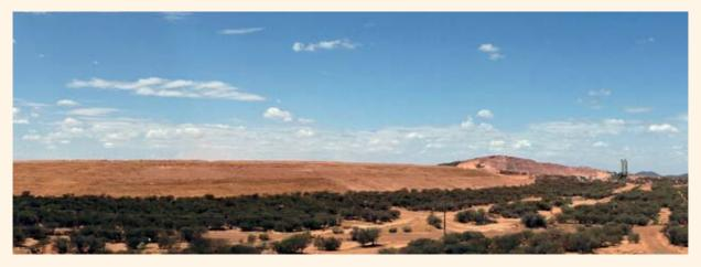
A panoramic view of the waste rock dump profiled, and with topsoiled batters ready for revegetation.
