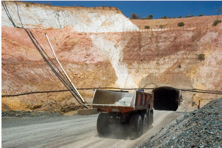
Decline to underground
