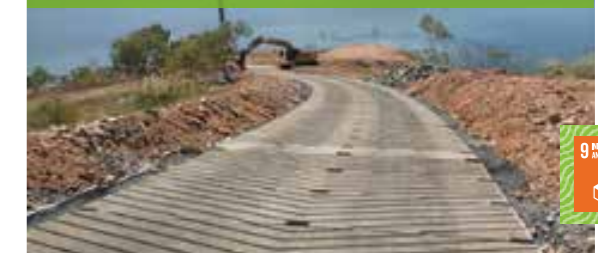
IMAGE: TSF access road, Dugald River, Australia.
