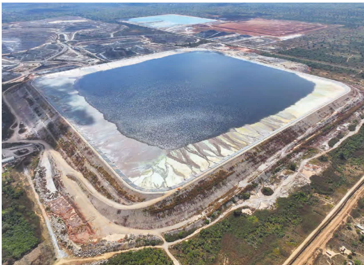
Figure 6: Aerial Image of Kinsevere TSF2
