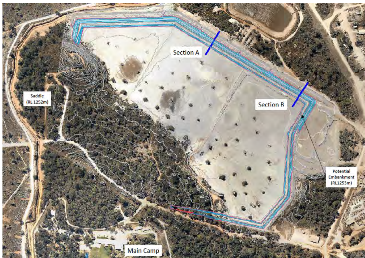
Figure 4: Aerial Overview of Kinsevere TSF1
