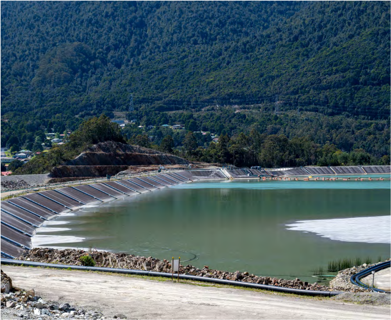
Figure 12: Rosebery 2/5 Dam TSF
