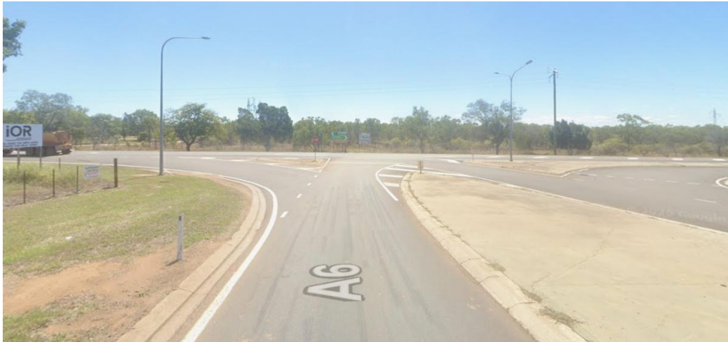
Figure 21: Flinders Highway southern approach to Flinders Highway/Gregory Developmental Road (Google Maps, March 2024)
