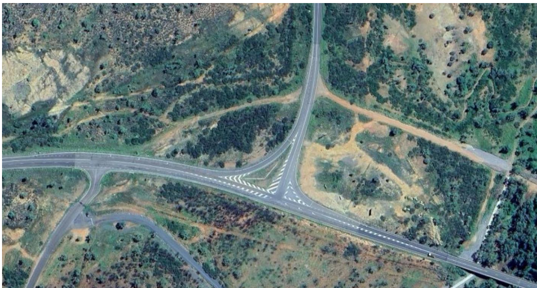
Figure 43: Aerial photography of Barkly Highway/Burke Development Road intersection location (www.google.com/maps, 2026)
