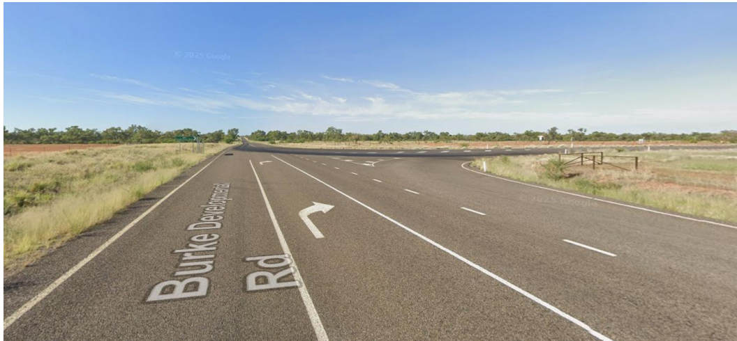
Figure 40: Northern Burke Development Road approach to the Burke Development Road/Dugald River Site Road intersection ( www.google.com/maps , 2026)
