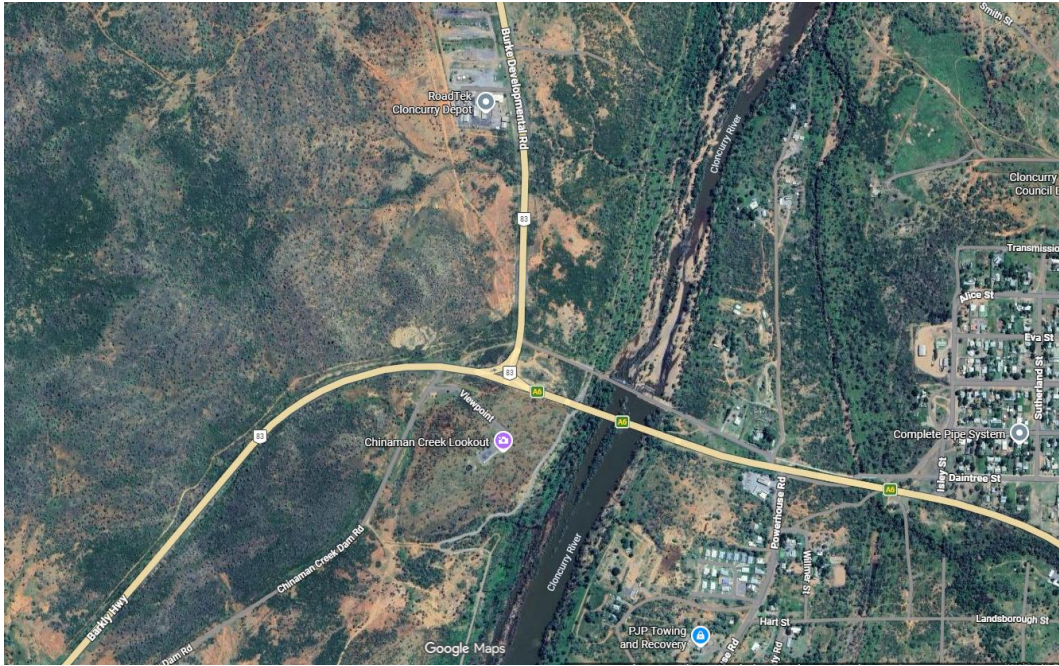
Figure 42.: Aerial photography of Barkly Highway/Burke Development Road intersection location (www.google.com/maps, 2026)
