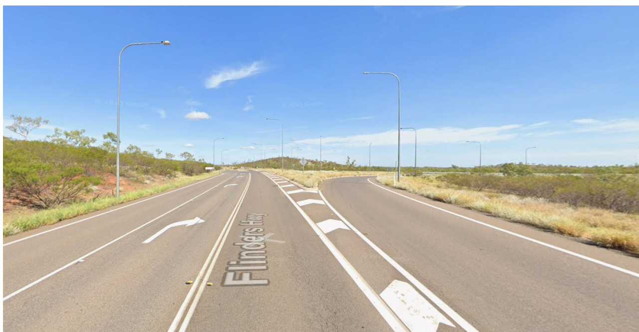
Figure 26: Eastern Flinders Highway approach to Flinders Highway/Andrew Daniels Drive Intersection (Google Maps, March 2025)
