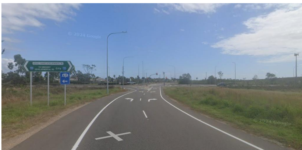
Figure 10: Bruce Highway exit lane southern approach to Hervey Range Developmental Road (Google Maps, March 2024)
