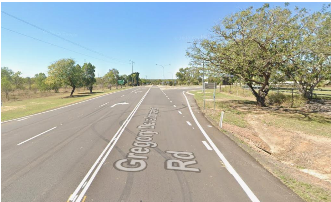
Figure 19: Gregory Developmental Road northern approach to Flinders Highway (Google Maps, March 2024)
