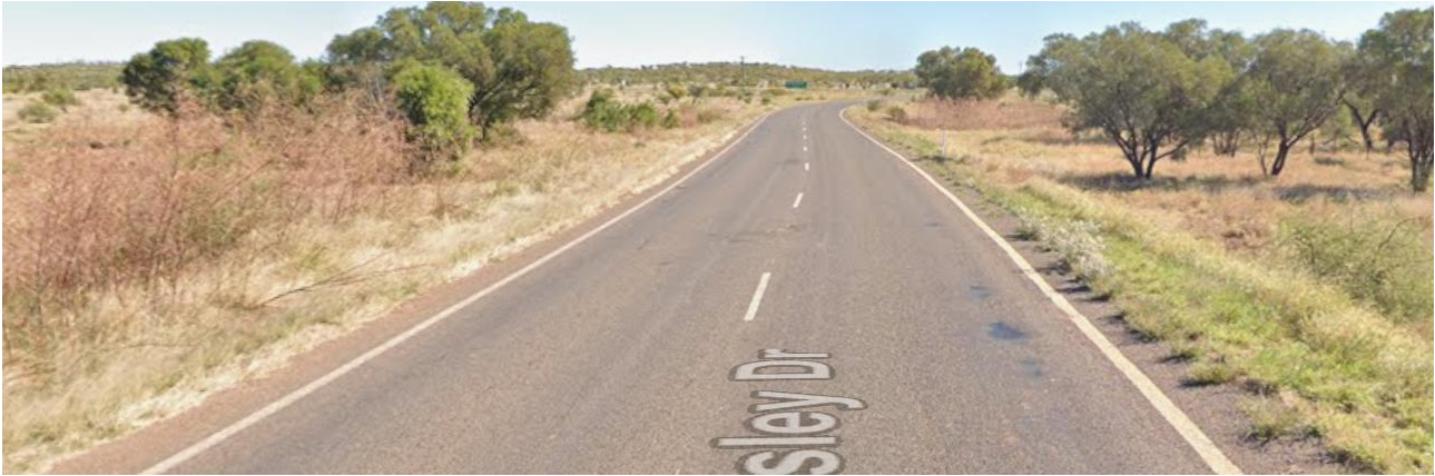
Figure 30: Hensley Drive looking west towards Burke Developmental Road (Google Maps, July 2023)
