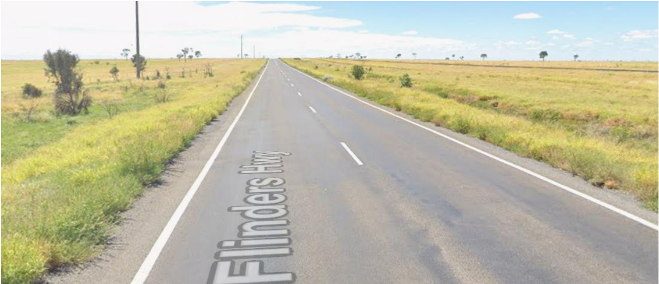
Figure 22: Flinders Highway looking west between Hughenden and Richmond (Google Maps, March 2025)
