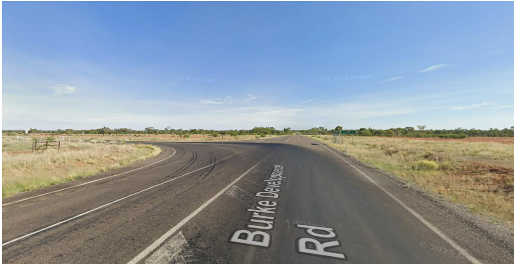
Figure 39: Southern Burke Development Road approach to the Burke Development Road/Dugald River Site Road intersection ( www.google.com/maps , 2026)
