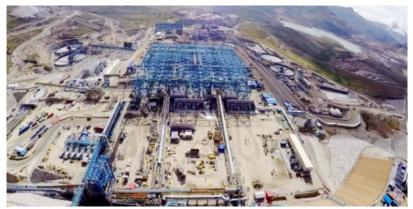
Dual train, conventional copper concentrator with 1.1m dry metric tpa output design capacity.
