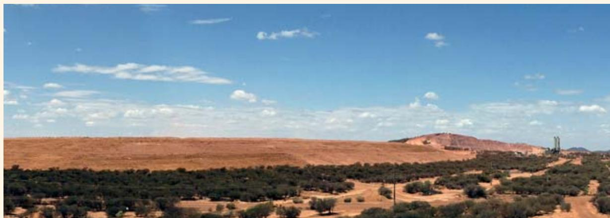
A panoramic view of the waste rock dump profiled, and with topsoiled batters ready for revegetation.
