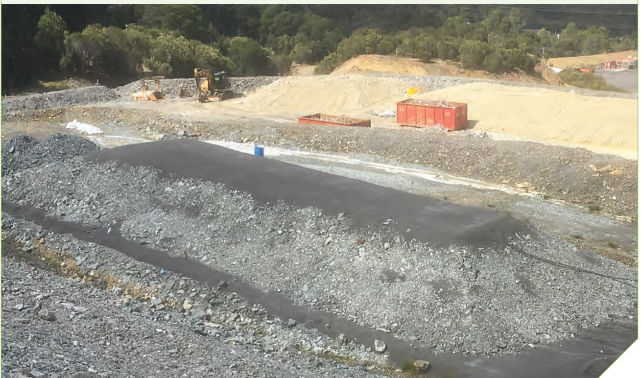
Image: Waste rock dump trial pad at Rosebery mine.
